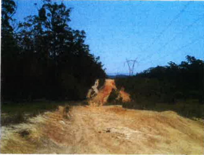
Figure 5 Formed road destroyed, now unusable by emergency vehicles
