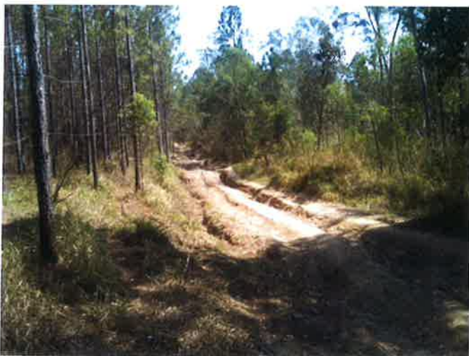
Figure 6 Fire Trail destroyed, used during wet weather
